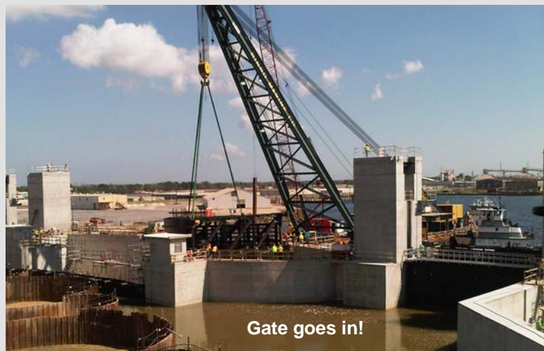
Gate is hoisted for placement
