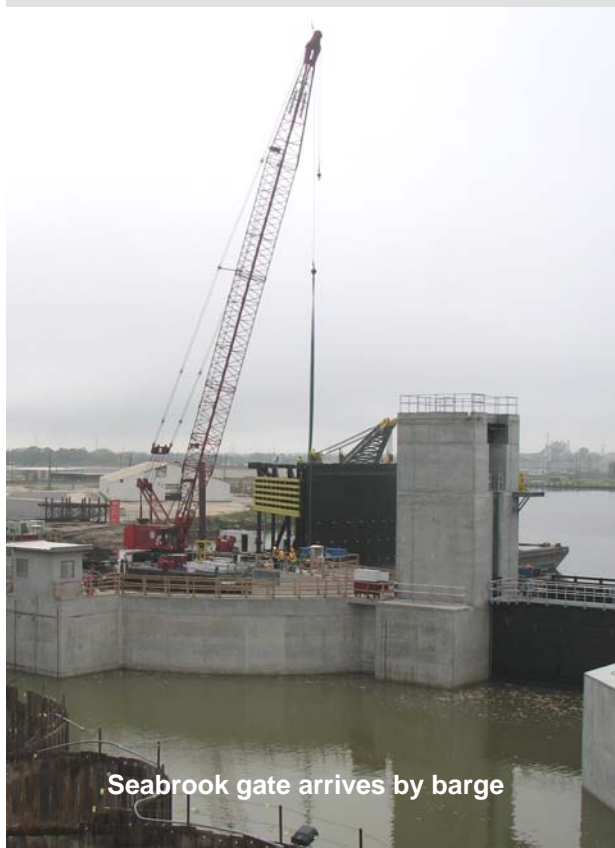
Gate is hoisted for placement
